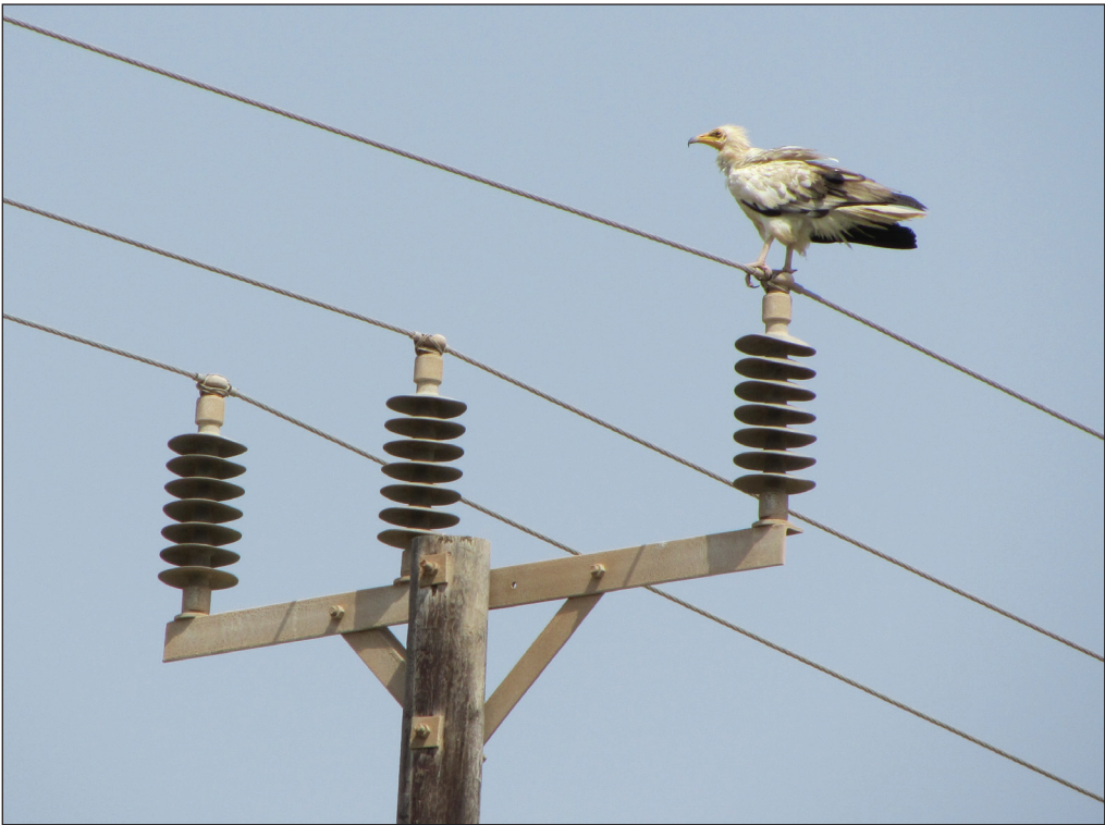
Plate 9. Egyptian Vulture Neophron percnopterus perched on electricity pylon, with vertical insulators above a horizontal crossbar, a design type that is considered dangerous in terms of electrocution risk, Masirah island, Oman. © Iyaylo Angelov
